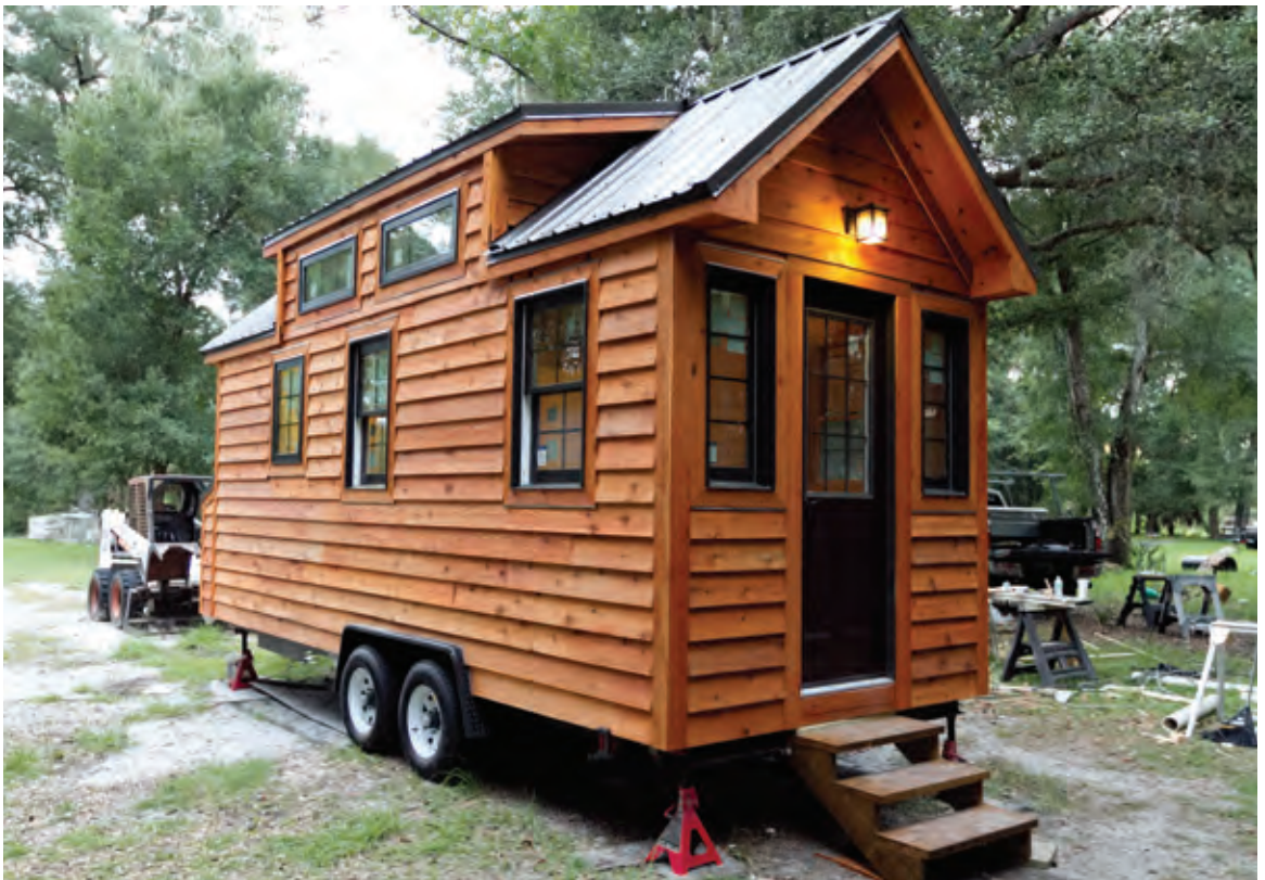
Trim and Siding Completed
