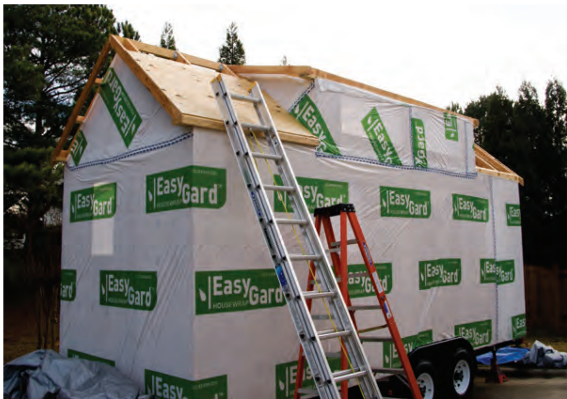
Roof Sheathing in Place
