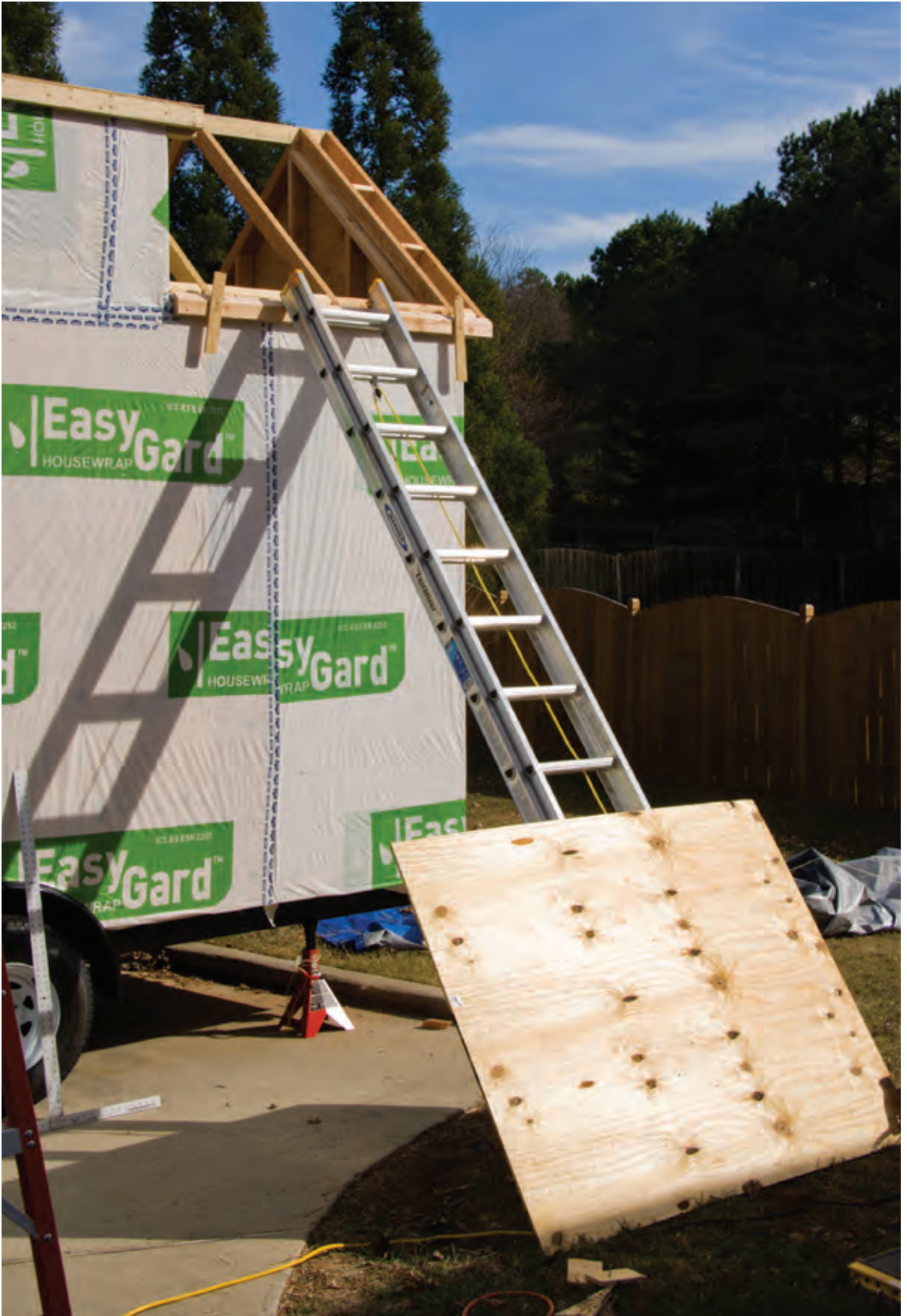
Roof Sheathing Ready to be Slid into Place
